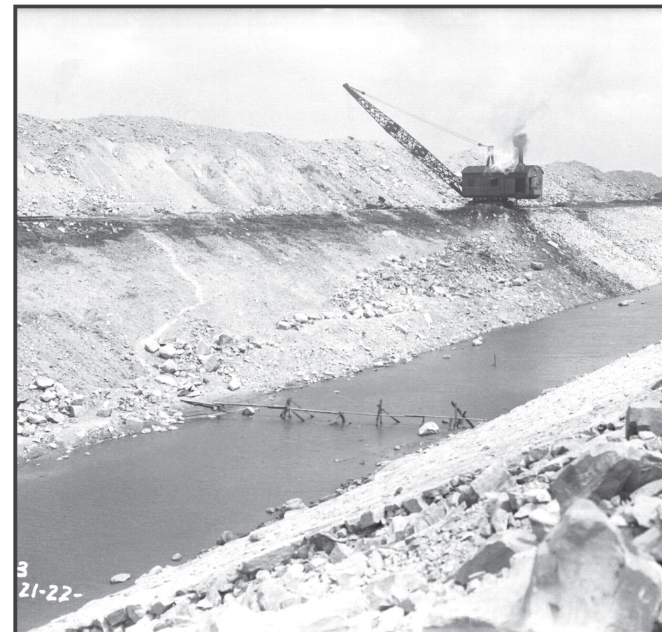
FIGURE 2: BUILDING THE CAL-SAG CANAL | Source: MWRD
