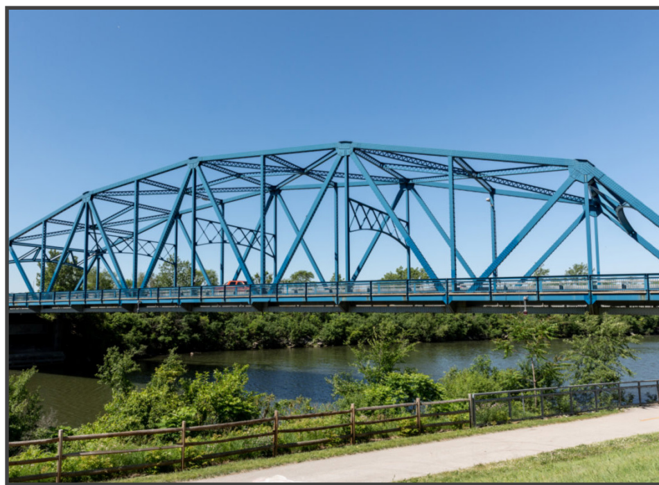
FIGURE 5: BRIDGE OVER THE CAL-SAG CANAL | Source: @Properties
